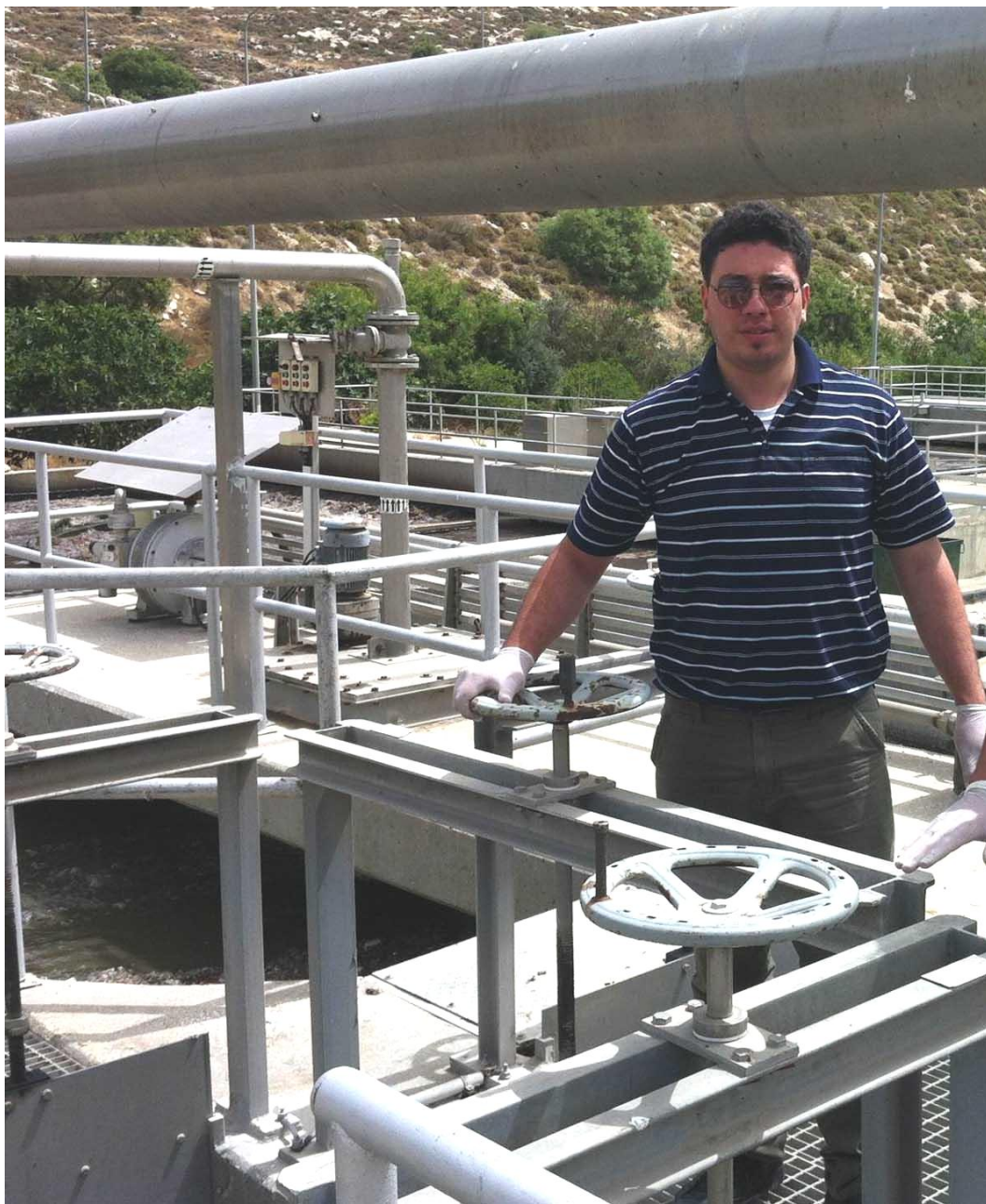
Photo 5: a side of Al-Bireh wastewater treatment station, during collecting samples of influent and effluent wastewater/ Al-Bireh /Palestine. (15 July, 2013)
