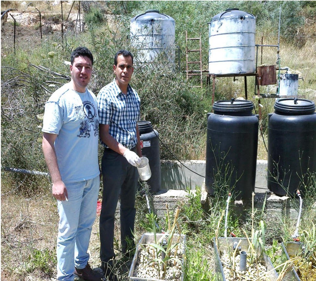
Photo 1: HSSFCW in operation, photo date (27/March, 2013)/ BZU/ Palestine
